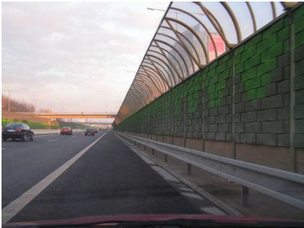
Figure 2.10 Noise barriers along the D1 motorway.
