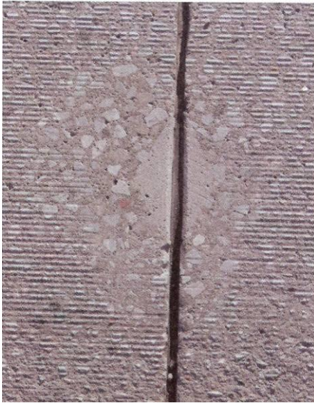
Figure 3.2 Example of reparation of a joint that shows the pattern (horizontal tight lines) after grinding the concrete road surface.
