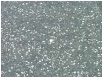
AB: Hot Rolled Asphalt:
